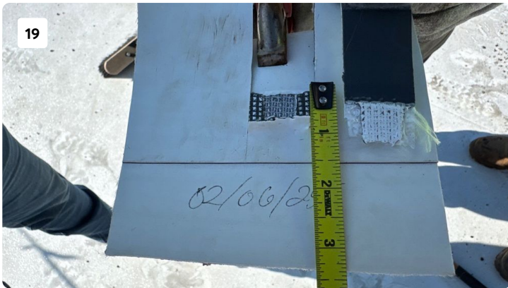
Weld pull test is good. material failed, the weld did not.
