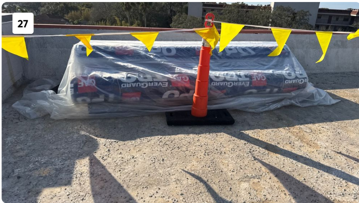
Rolls of .60mil GAF TPO Smooth are onsite
