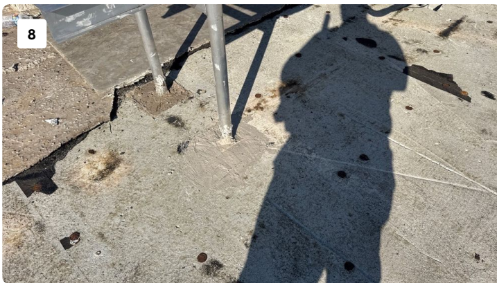
Lightweight concrete was back filled at all legs
