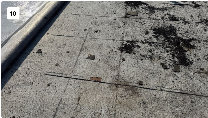
The lightweight concrete is in good condition
