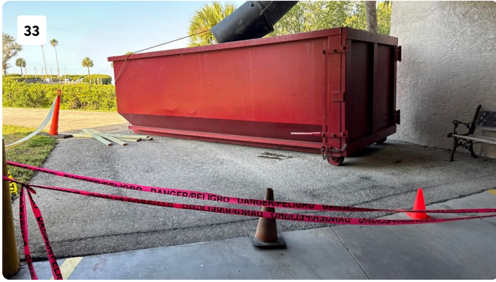
Dumpster staging area
