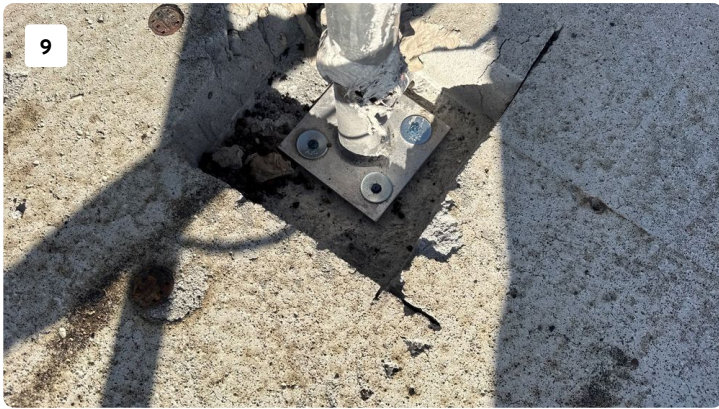
Roof stands are properly secured.
