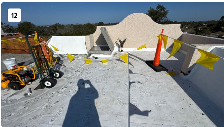
Approx. 20sq of roofing has been laid up.
