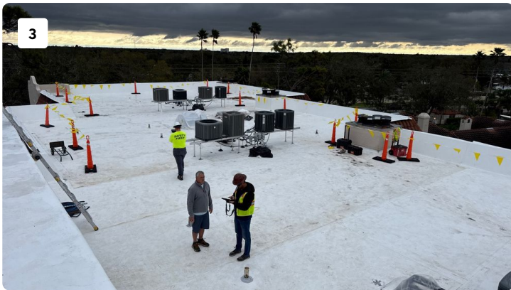
Roof Overview Images
