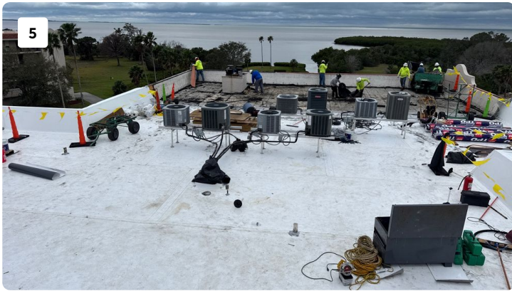
Roof Overview Images: Approx. 90% has been laid up as of 2-20-25 @ 8:30am
