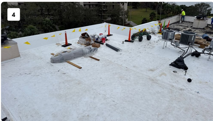
Roof Overview Images
