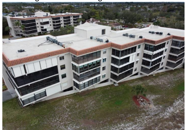
4 Left Side of Building #504
