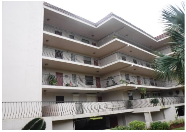
2 Right Side of Building #504
