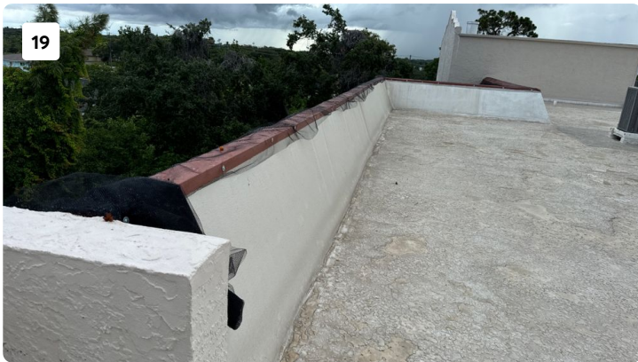
new coping cap all the way around
