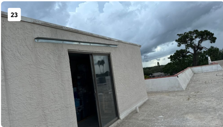
new gutters around the penthouse roofs.
