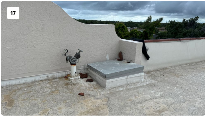
roof hatches will stay and be flashed in.
