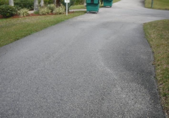
109 Building #504 Pavement Overview
