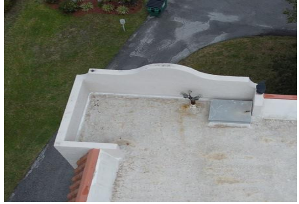
78 Building #504 Roof Hatch Overview
