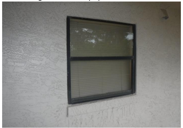
62 Bldg. #502 Unit Windows Overview
