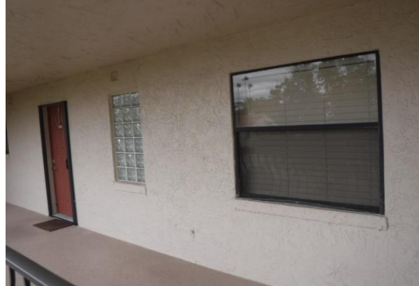
118 Building #504 Unit Doors and Windows
