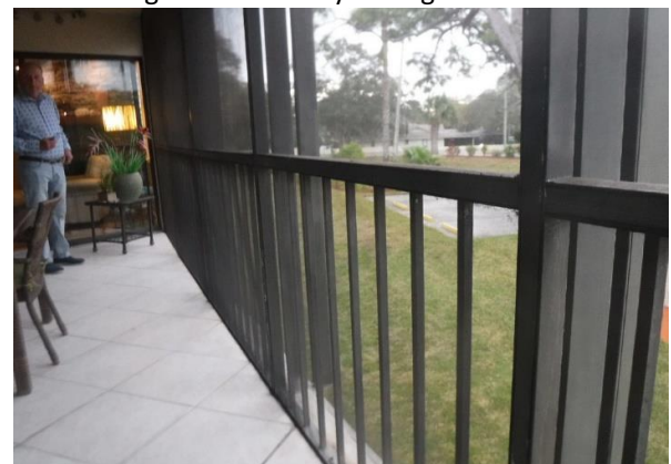
40 Bldg. #502 Balcony Railing Overview
