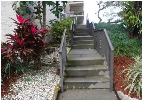
111 Building #504 Sidewalk Overview
