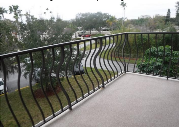
103 Building #504 Walkway Railings Overview
