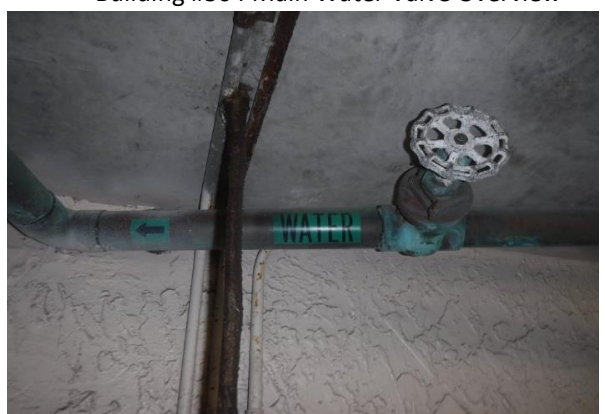
98 Building #504 Plumbing Chase Overview
