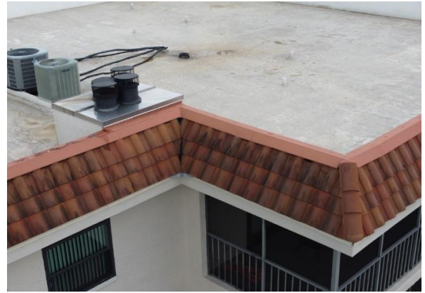
10 Bldg. #502 Tile Roofing Overview
