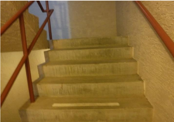
21 Bldg. #502 Stairway Paint Overview
