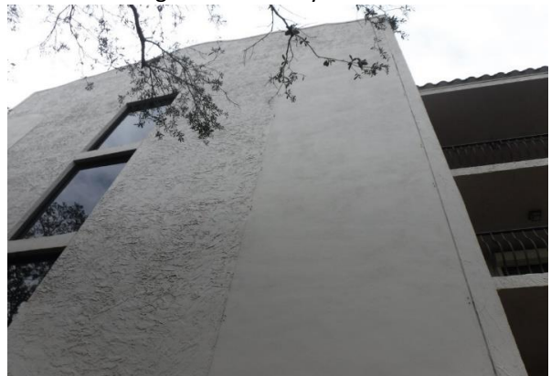
82 Building #504 Building Paint Overview
