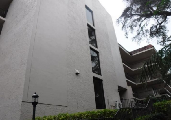
65 Bldg. #502 Building Windows Overview
