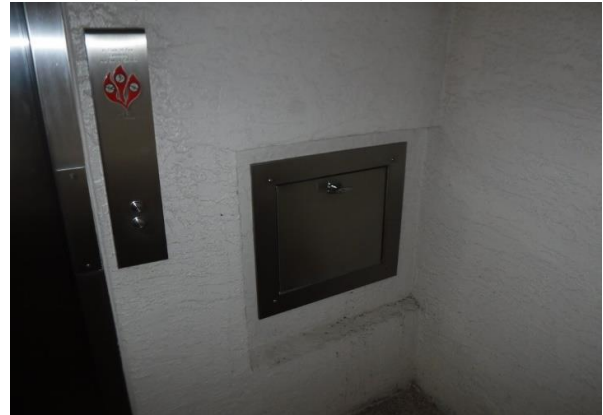
56 Bldg. #502 Trash Chute Overview
