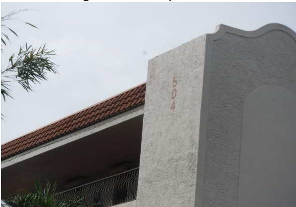
81 Building #504 Building Paint Overview
