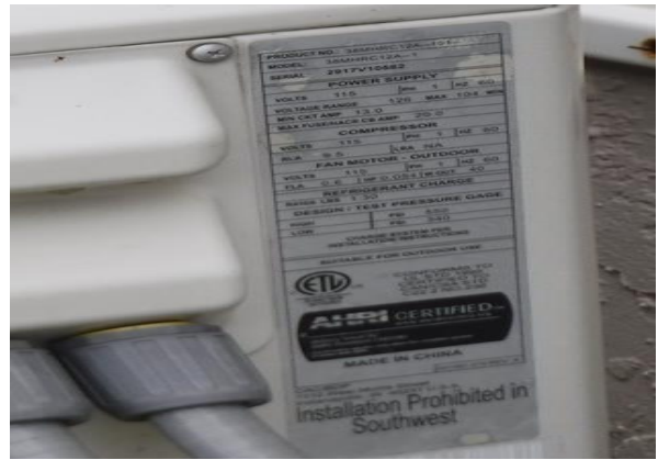
116 Building #504 HVAC Split Data Plate
