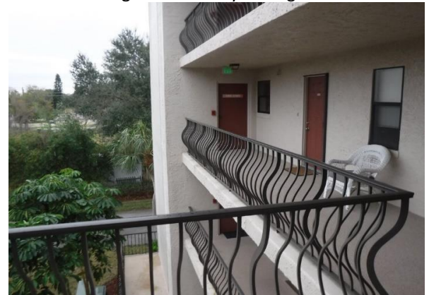
104 Building #504 Walkway Railings Overview
