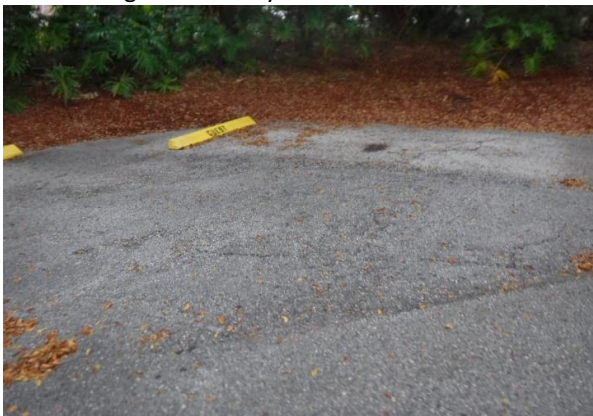
45 Bldg. #502 Pavement Overview
