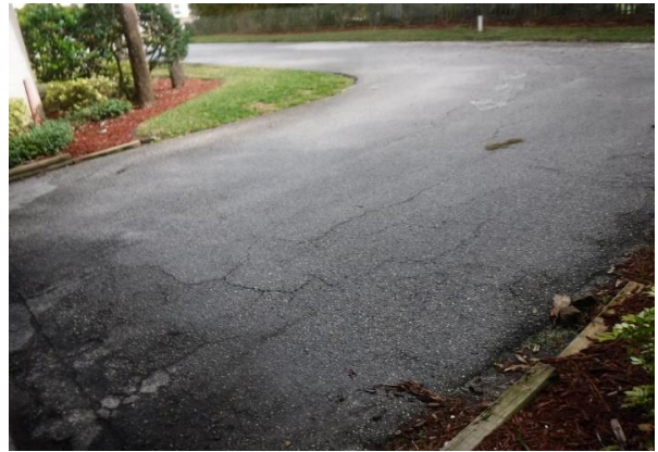
108 Building #504 Pavement Overview
