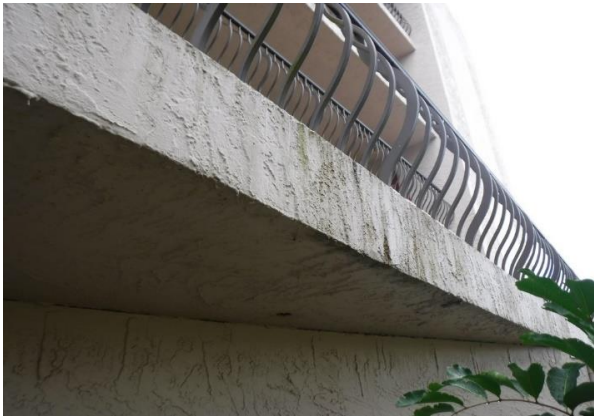
83 Building #504 Building Paint Overview
