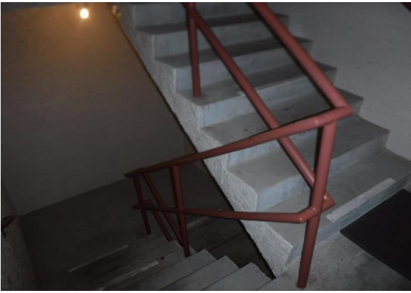
99 Building #504 Stairway Railings Overview
