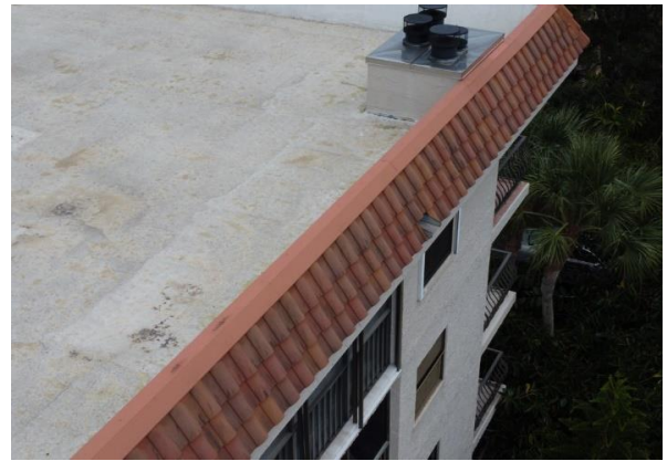
76 Building #504 Tile Roofing Overview
