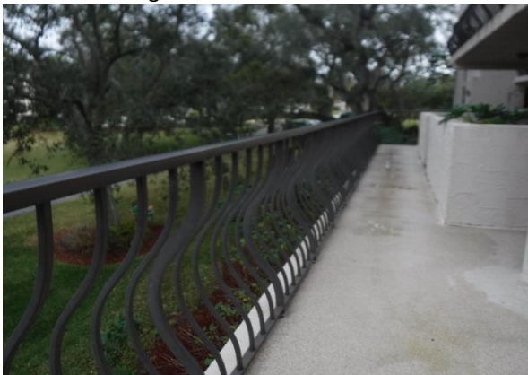
79 Building #504 Walkway Paint Overview
