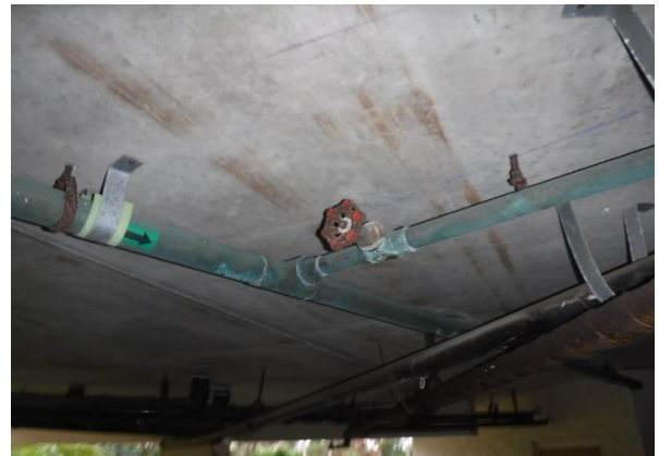
34 Bldg. #502 Plumbing Chase Overview
