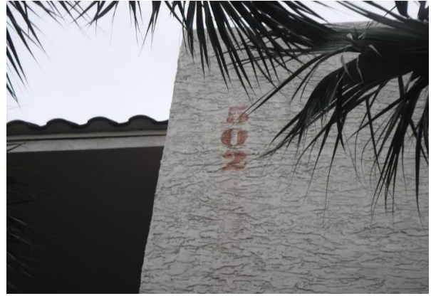
18 Bldg. #502 Building Paint Overview
