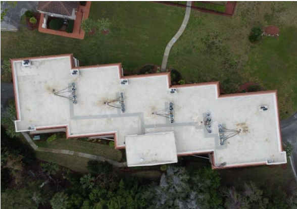
5 Bldg. #502 TPO Roofing Overview
