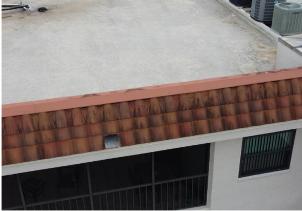
11 Bldg. #502 Tile Roofing Overview
