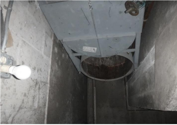
57 Bldg. #502 Trash Chute Overview
