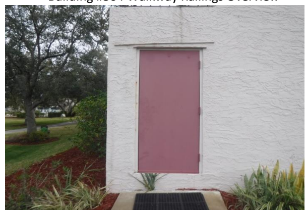
106 Building #504 Utility Doors Overview
