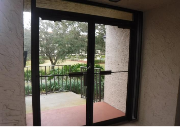
107 Building #504 Double Glass Doors Overview
