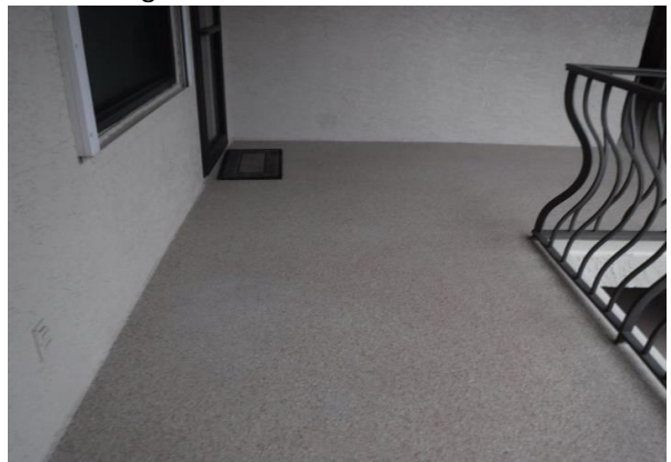
14 Bldg. #502 Walkway Paint Overview
