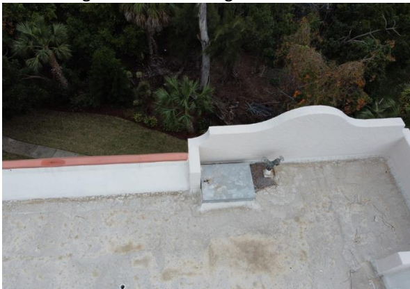
13 Bldg. #502 Roof Hatch Overview
