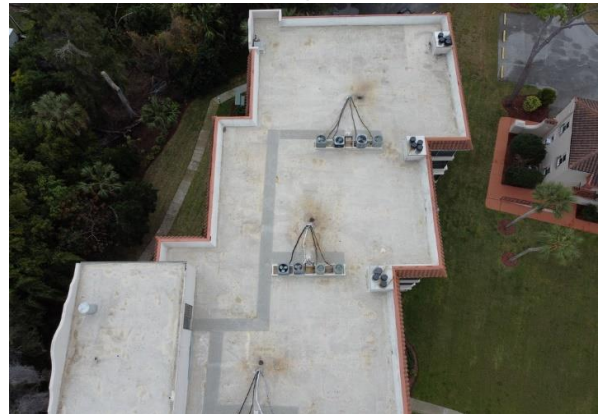
6 Bldg. #502 TPO Roofing Overview
