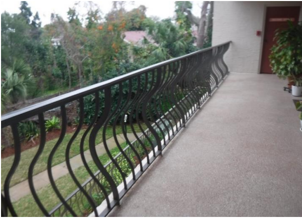
41 Bldg. #502 Walkway Railing Overview
