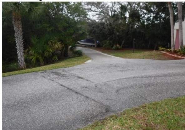
47 Bldg. #502 Pavement Overview
