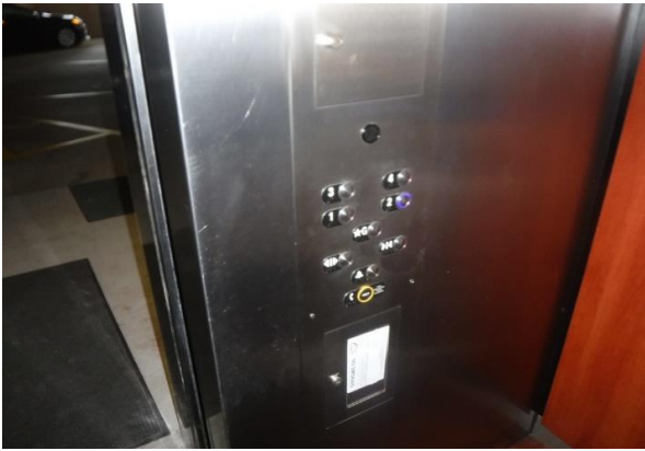
25 Bldg. #502 Elevator Cab Overview
