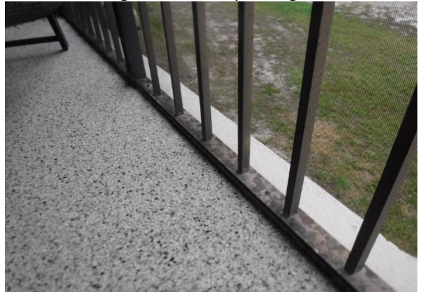
102 Building #504 Balcony Railings Overview
