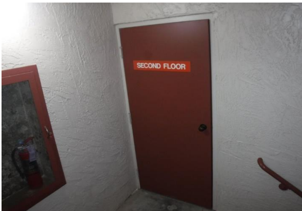
23 Bldg. #502 Stairway Paint Overview
