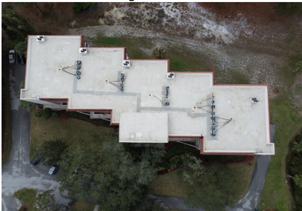
71 Building #504 TPO Roofing Overview
