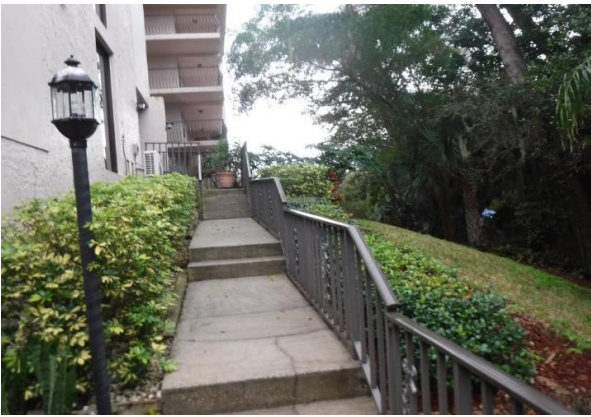
49 Bldg. #502 Sidewalks Overview
