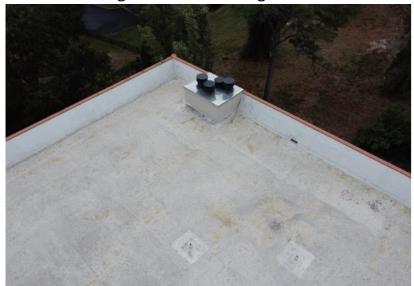
74 Building #504 TPO Roofing Overview
