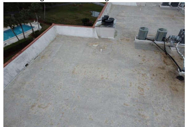
8 Bldg. #502 TPO Roofing Overview
