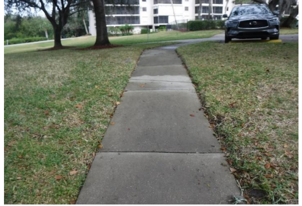
110 Building #504 Sidewalk Overview
