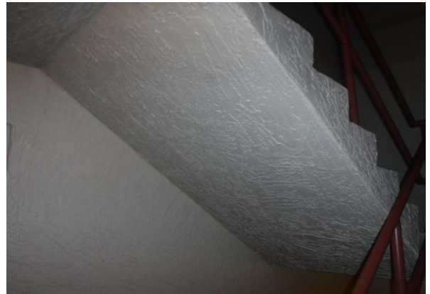
22 Bldg. #502 Stairway Paint Overview
