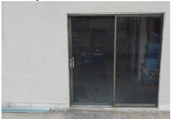
64 Bldg. #502 Rooftop Slider Overview
