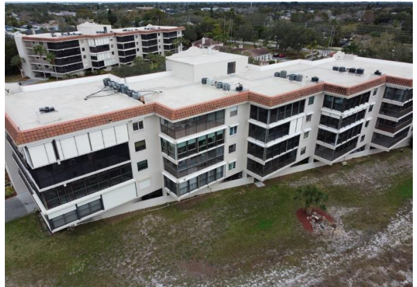
70 Left Side of Building #504
