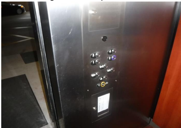
87 Building #504 Elevator Cab Overview
