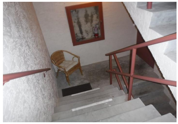
100 Building #504 Stairway Railings Overview
