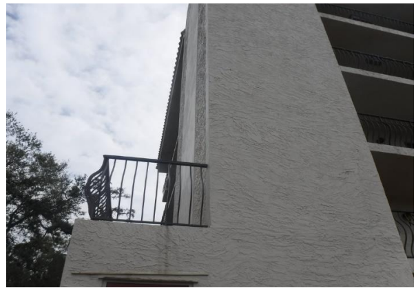
84 Building #504 Building Paint Overview
