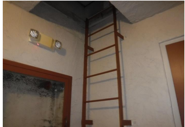
86 Building #504 Stairway Paint Overview
