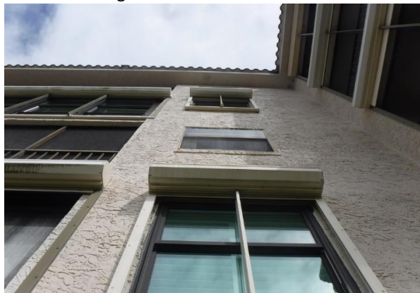
119 Building #504 Unit Windows
