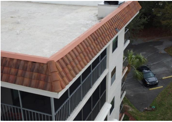
9 Bldg. #502 Tile Roofing Overview
