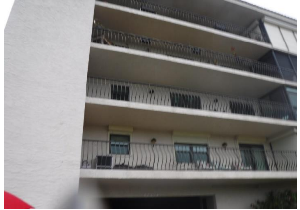
42 Bldg. #502 Walkway Railing Overview
