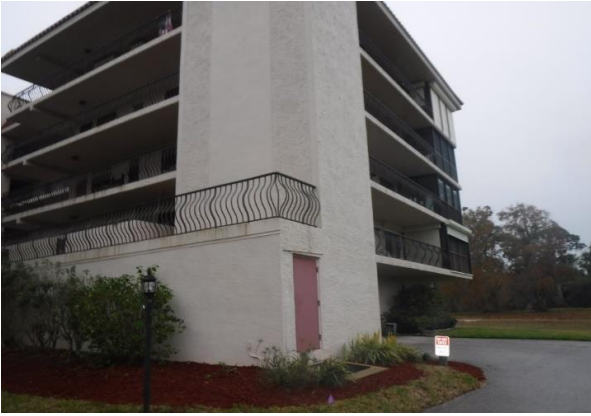
17 Bldg. #502 Building Paint Overview
