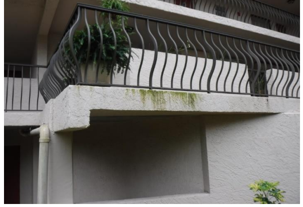
20 Bldg. #502 Building Paint Overview
