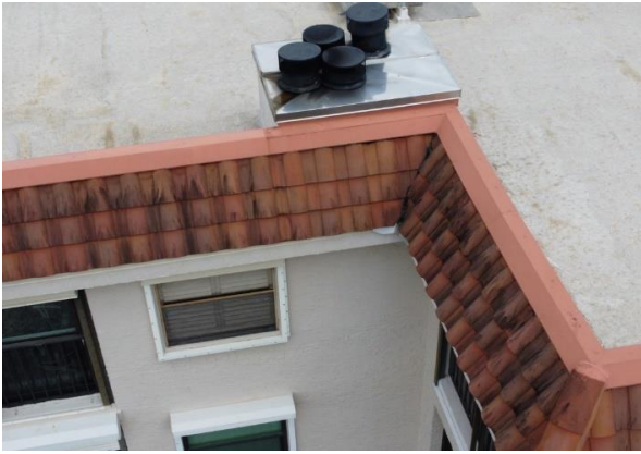
75 Building #504 Tile Roofing Overview
