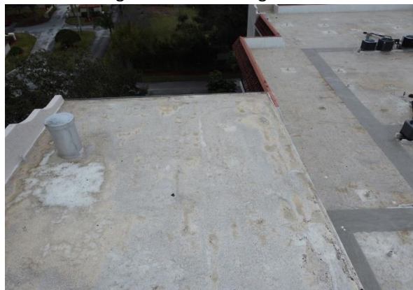
73 Building #504 TPO Roofing Overview
