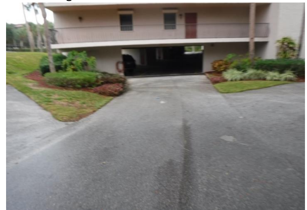
46 Bldg. #502 Pavement Overview
