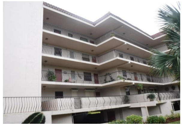
2 Right Side of Building #502
