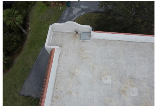
72 Building #504 TPO Roofing Overview
