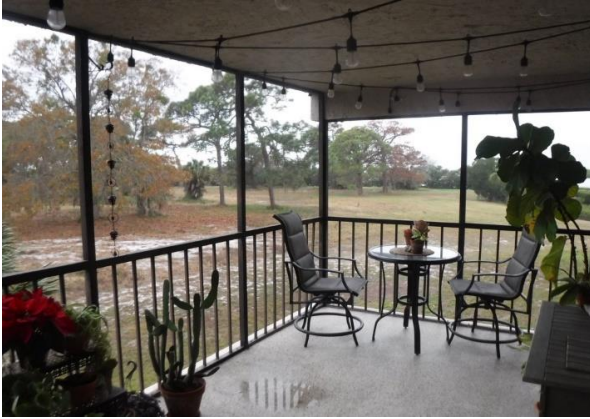
101 Building #504 Balcony Railings Overview
