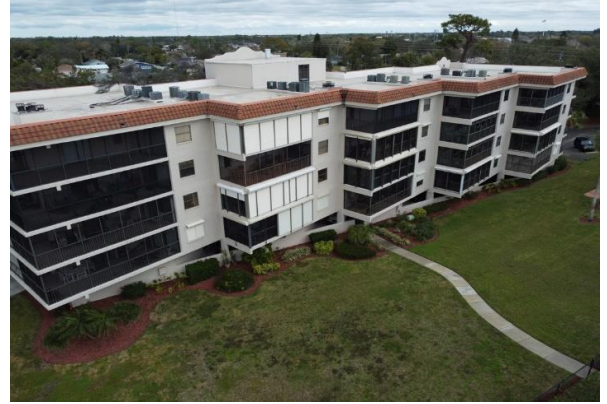
4 Left Side of Building #502
