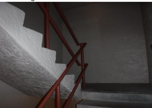
37 Bldg. #502 Stairway Railing Overview
