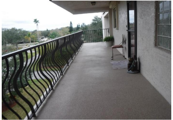
80 Building #504 Walkway Paint Overview
