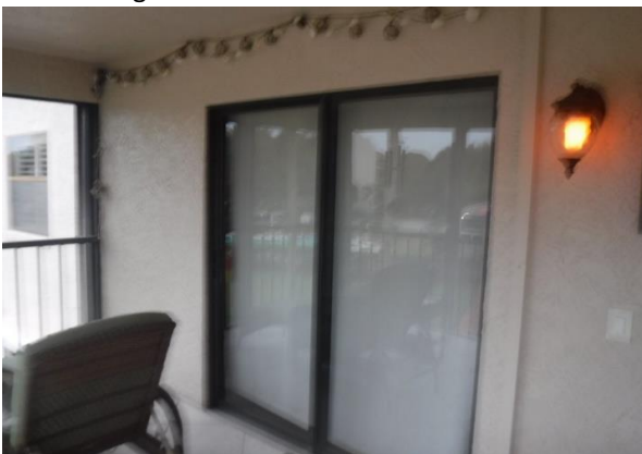
63 Bldg. #502 Unit Sliders Overview
