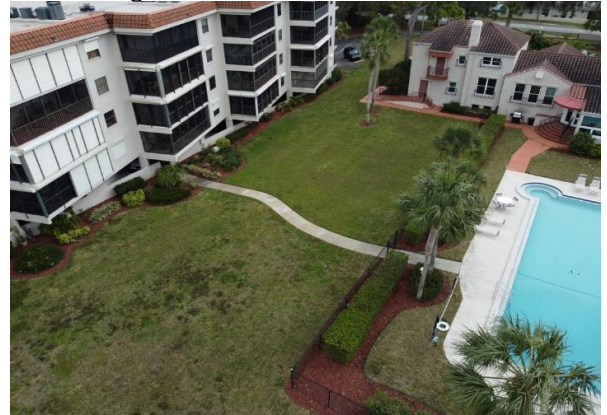
48 Bldg. #502 Sidewalks Overview
