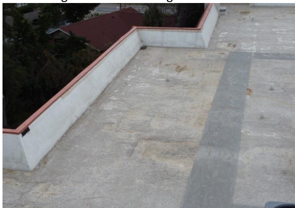
7 Bldg. #502 TPO Roofing Overview
