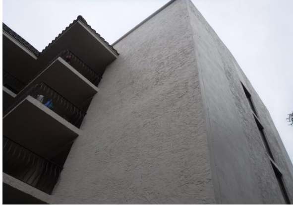
19 Bldg. #502 Building Paint Overview
