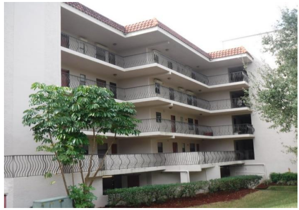
68 Right Side of Building #504
