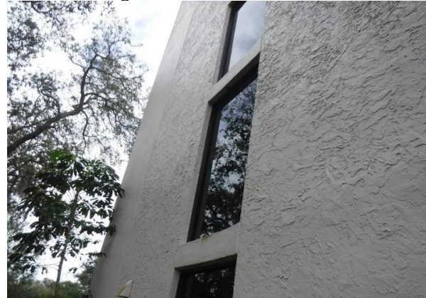
122 Building #504 Building Windows
