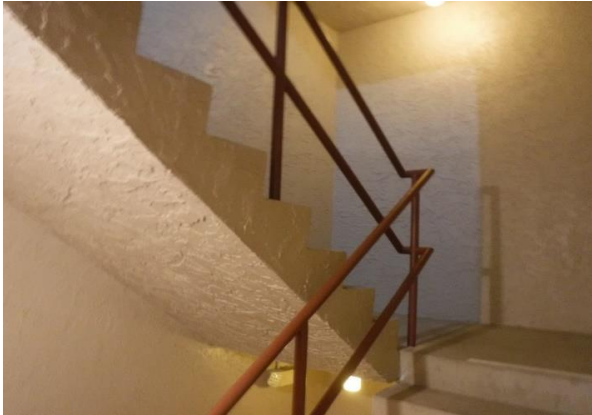
85 Building #504 Stairway Paint Overview
